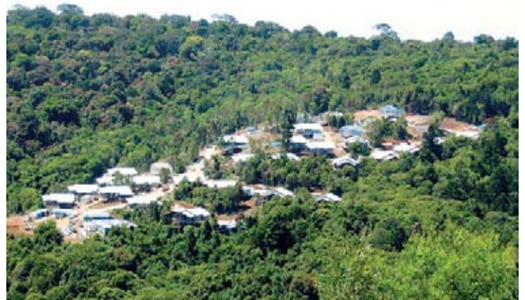
An aerial photo of O'Reilly's Mountain Bowers villas.
